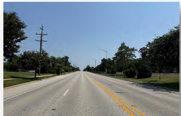
Northwest Highway at the crossing location
